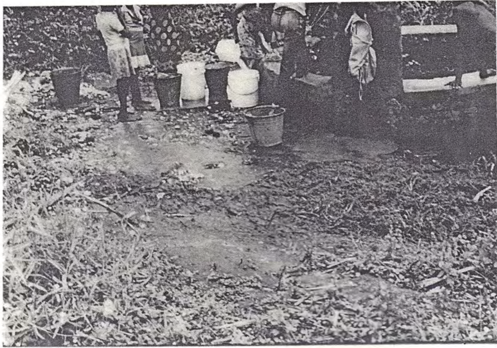
P.3. Bad drainage around well
