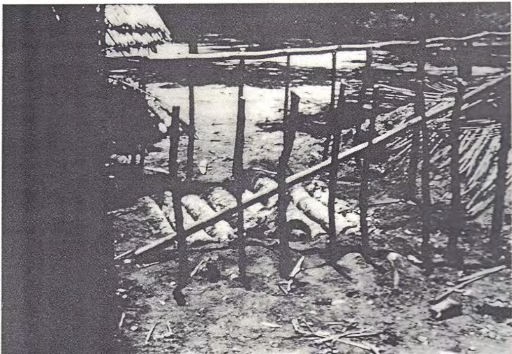
P.8. Latrine (open pit type) under construction.
